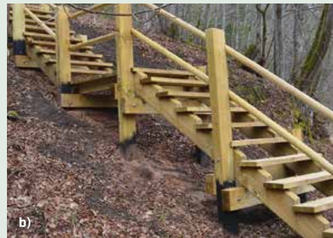
Fig. 15.12. Stairway on slope (A), raised above the ground on dug-in wooden posts (B). Photo: S. Ikauniece.
