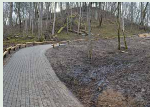
Fig. 15.15. One should definitely avoid the construction of large trails with heavy material on slopes, as part of the habitat is thus irreversibly destroyed and erosion is promoted like here. Photo: S. Ikauniece.
