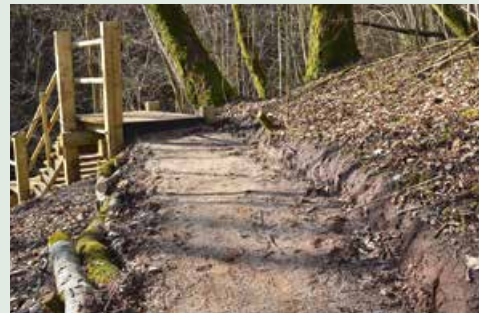
Fig. 15.13. A small walkway (~0.7 m wide), slightly dug into the slope. The edge of the trail has been fixed with logs of small dimension, preventing potential erosion. Photo: S. Ikauniece.
