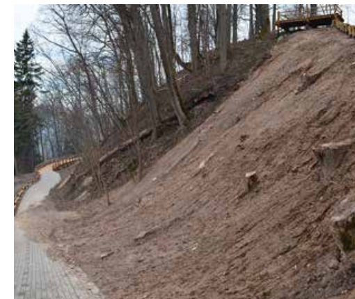
Fig. 15.7. Erosion processes in Gauja National Park along the "Serpentine road" ("Serpentina ceļš"). Photo: S. Ikauniece.
