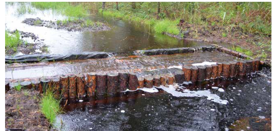
Fig. 13.6. Wooden dam in Estonia. Photo: S. Ikaunieca
