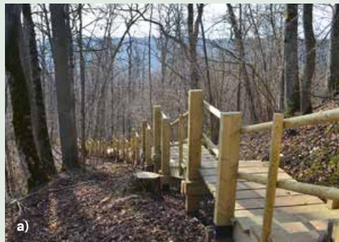
Fig. 15.12. Stairway on slope (A), raised above the ground on dug-in wooden posts (B). Photo: S. Ikauniece.
