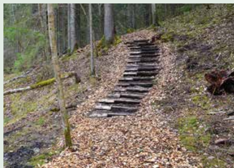
Fig. 15.14. A stairway of wooden planks built on a slight slope. Wooden chips were used for the trail and adjacent area to the stairway. Photo: S. Ikauniece.
