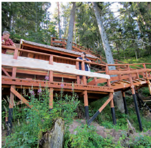
Fig. 11.31. Stairs and a sightseeing platform at Dauģēni outcrop. Photo: I. Čakare.
