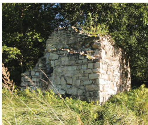
Fig. 2.5. Buildings, for whose construction dolomite pieces are used, are often seen in the surroundings of exposed carbonate rocks (Baltiņi farm house in Priekulji Municipality). Photo: I. Čakare.
