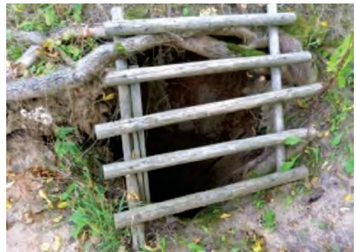
Fig. 12.9. Ciruliši Cave, a vertical cave (a hole in the ground below which there is a wide cave room), closed with a horizontal wooden grille which is situated too close to the ground, thus making bat entry difficult. Photo: I. Čakare.
