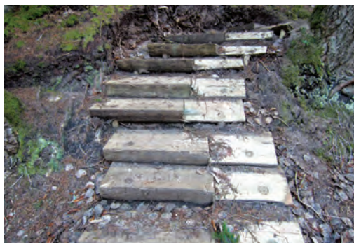
Fig. 11.29. Wooden plank stairs at Liči-Laņģi Cliffs enable the creation of a complex configuration, because each step is separately fixed with wooden pegs. Wood is a material that wears out rapidly, but each of these steps can be restored separately. However, such steps tend to bend and slide out of place. Photo: I. Čakare.
