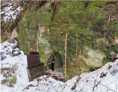
Fig. 12.13. Long abandoned cellar caves in Ligatne. Only the support wall on the left remains. Entrance doors and their mountings are missing. Photo: I. Čakare.
