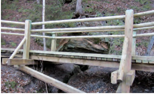
Fig. 11.32. Footbridge over the spring at Liči-Lanģi Cliffs. Photo: I. Čakare.
