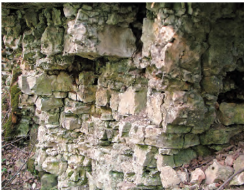
Fig. 10.7. Structure of calcareous outcrops is characterised by vertical and horizontal cracks. Outcrop in Korkuļi ravine. Photo: A. Priede.
