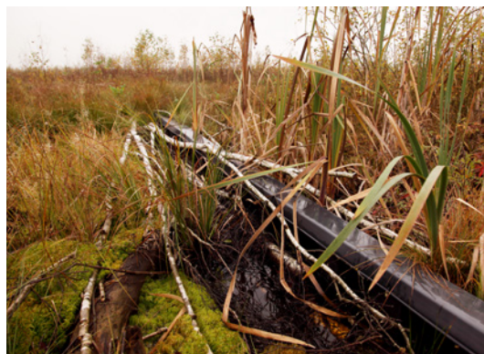
Fig. 10.32. A plastic piling dam in extracted peatland in Žuvintas Biosphere Reserve in Lithuania. Photo: M. Pakalne.
