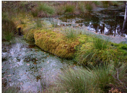
Fig. 10.26. Hand built wooden dam, built around 1997, after a longer time completely overgrown with Sphagnum spp. and Eriophorum vaginatum . Teiči Bog, the photo is taken in 2013. Photo: M. Priedēna.
