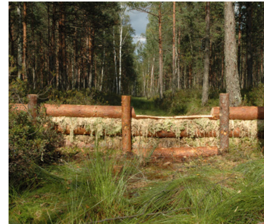
Fig. 10.28. Log dam packed with Sphagnum spp., Rāksala in Teiči Bog in 2004. Photo: J. Jātņieks.
