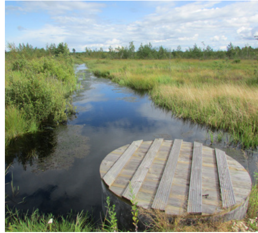
Fig. 2.14. Rewetted bog in the "Ādaži" Protected Landscape Area. In raising the water level a water flow regulator was built. The photo was taken in 2014, around two years after restoration. Photo: A. Priede.
