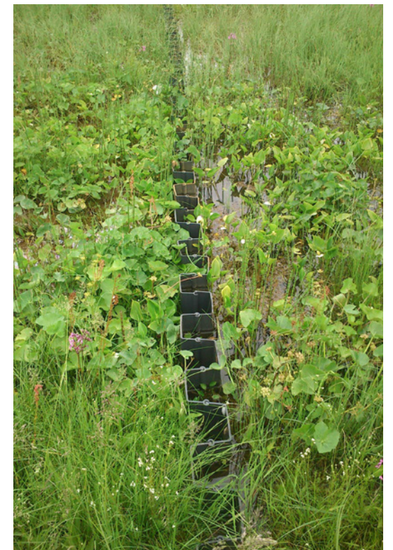
Fig. 15.16. A dam made of a corrugated plastic wall in a rich fen in Lithuania. Photo: G. Eriņš.
