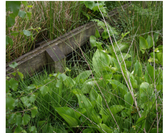
Fig. 15.15. A wooden dam made of planks in a rich fen in Germany. Photo: M. Priedēna.
