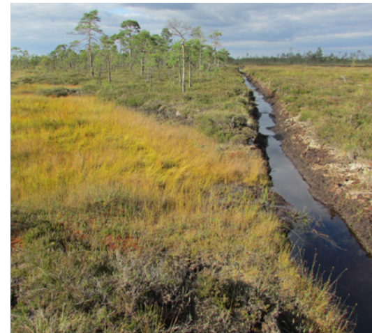
Fig. 10.47. A recently dug ditch in Aizkraukle Bog along the edge of the newly planned peat milling field and along the edge of the intact bog. To diminish the undesirable impact on the bog, the waterproofing membrane should be installed parallel to the ditch in the early stage of draining, prior to significant reduction of the water table in the planned peat extraction site. Photo: A. Priede.
