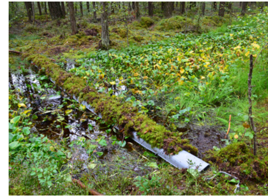
Fig. 10.34. A plastic dam masked with moss cover to encourage its faster overgrowing and integration in the surroundings. Kamanos Strict Nature Reserve in Lithuania. Photo: S. Ikauniece.
