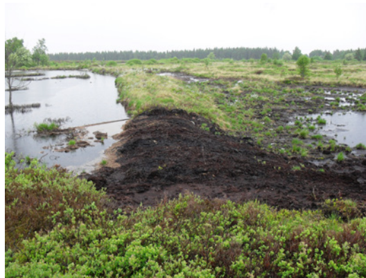
Fig. 10.60. A dyke built of peat in a post-harvested peatland on slope. The photo is taken in a restored post-harvested peatland in Germany. Photo: K. Lapiņš.
