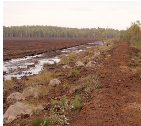
Fig. 10.46. Waterproofing wall made from plastic sheeting, covered by the peat dyke along the outer edge of extracted peatland in Aukštumala Bog in Lithuania. Photo: M. Pakalne.
