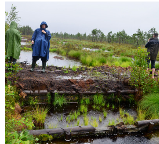
Fig. 10.30. Wooden dam filled with peat in a bog in Estonia. Photo: S. Ikauniece.
