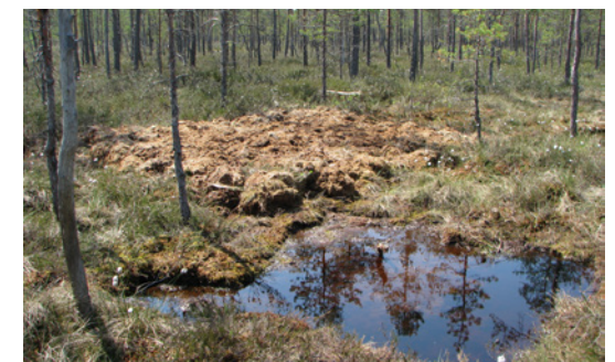
Fig. 10.37. Hand-built peat dam in Aklais Bog (in 2013). Peat has been dug out from the bog surface near the dam. Photo: A. Priede.
