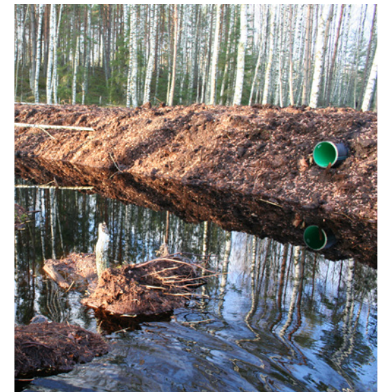
Fig. 10.44. Peat dyke (large dam) in Great Ķemeri Mire. The purpose of the dam is to keep the water level high in the extracted peatland upstream of the dam. To adjust the water level, a pipe is built in. Photo: A. Liepa.
