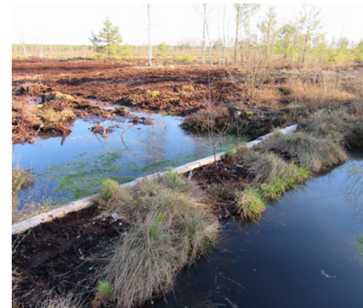
Fig. 10.29. Wooden dam of logs, upstream of the dam packed with peat, Viru Bog in Estonia. Photo: A. Priede.
