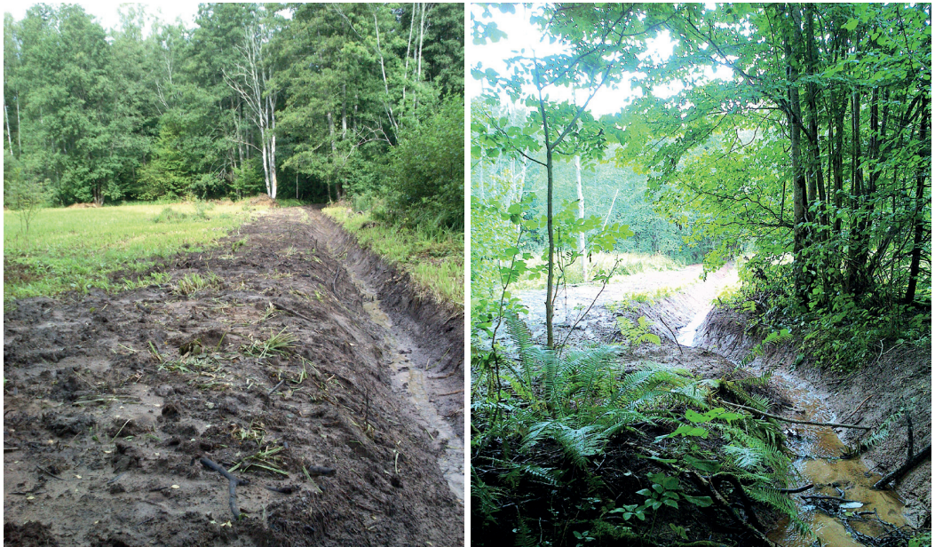
Fig. 14.5.2. A shallow ditch hand-dug in the first half of the 20th century is cleaned in Dāvidpļava. The removed soil has been spread out along the edge of the ditch. The vegetation there will recover in a few years. Photo: Slitere National Park archive.
