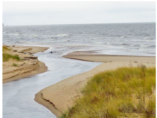
The renewed area is very unstable and will only last until the next storm, after which the activity must be repeated. R. Kurliņupe. Photo: G. Rubenis.
