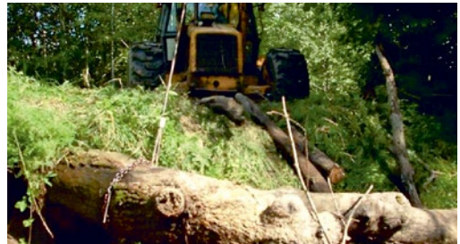
Large dimension log removal with power lift. R. Vitrupe. Photo: A.V.Urtāns.
