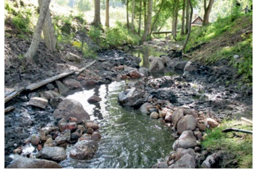
Fig 17.33. Channel narrowing. Sediment filled shallow channel stretch with negligible flow (1) is narrowed using stone riprap. Renewed flow scours sediments and re-creates diverse microhabitats suitable for salmonids (2). Kärji fish hatchery. Photo: A. V. Urtans
