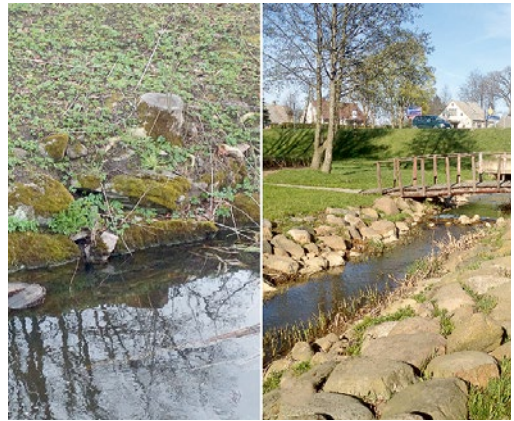
Fig. 17.31. Stones strengthen the riverbank against erosion, while also creating suitable habitats for aquatic and shore animals (1). The River Lazdupe in Ranka. Photo: L. Urtāne. Strengthening of riverbanks for rivers located in an urban environment River Stulpa in Lithuania is also used as a landscape design element and blue infrastructure. The amount of stones placed on the riverbank is greater than is needed for its strengthening (2). Photo: A. V. Urtāns.
