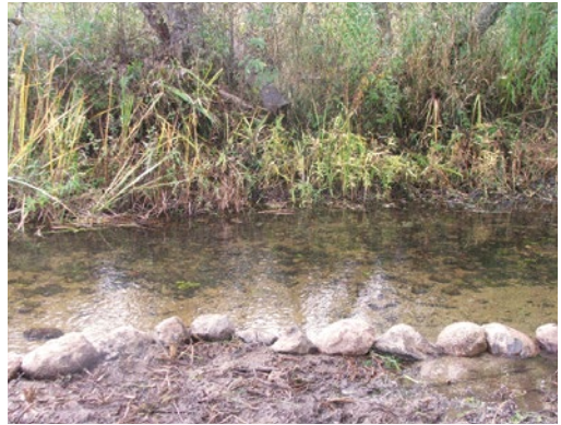
Area behind the stone line starts to overgrow with grasses and becomes stabilised. Method is applicable for small streams, which due to bank erosion have become wide and shallow. Photo: L. Urtāne.
