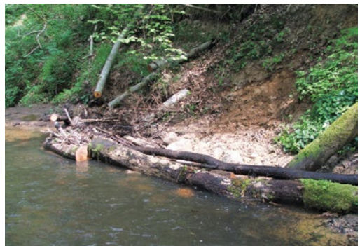
Fig. 17.32 Bank stabilisation undertaken to halt bank erosion and falling of an oak into the river (1). Eroded bank stabilised with stone riprap and additionally wooden trunks to promote bank revegetation (2). R. Kauliņa. Photo: A. V. Urtāns.
