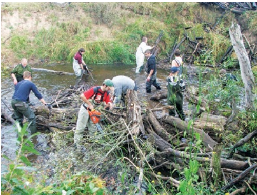
Removal of a log jam hindering water flow. R. Palsa. Photo: L. Urtāne.
