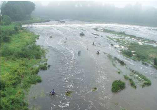
Workers standing across the river and using flow peculiarities, direct compacted macrophytes downstream to temporary storage area. R. Venta. Photo: L. Urtāne.
