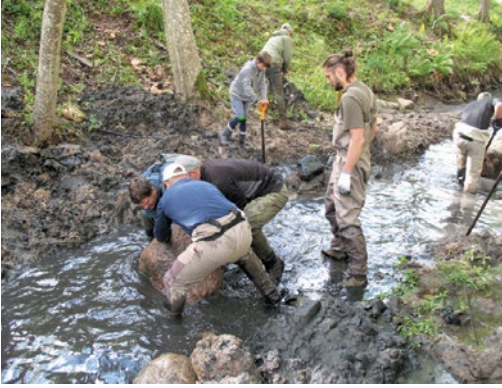
Narrowing of the channel to increase stream velocity, to scour sediments and reopen the gravel bottom. Photo: A. V. Urtāns.
