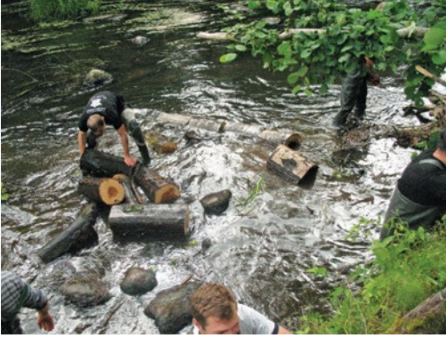
In cases, when removal of excessive timber logs is done manually, they are sawn in dimensions that can be lifted manually. R. Svētupe. Photo: L. Urtāne.
