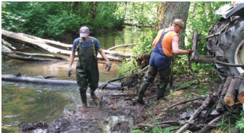
Large dimension log removal with wheel tractor. R. Kauliņa. Photo: L. Urtāne.
