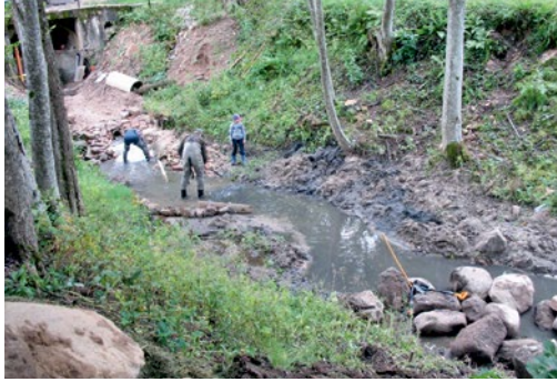
Fig 17.33. Channel narrowing. Sediment filled shallow channel stretch with negligible flow (1) is narrowed using stone riprap. Renewed flow scours sediments and re-creates diverse microhabitats suitable for salmonids (2). Kärji fish hatchery. Photo: A. V. Urtans
