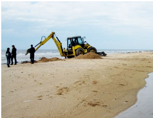
Excavated sand sediments are disposed nearby. R. Kurliņupe. Photo: G. Rubenis.
