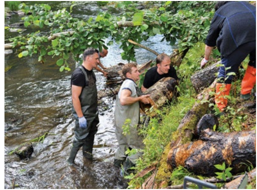
Timber logs are lifted and stored above the high water line. In rivers with steep banks it is a time and effort consuming activity. R. Svētupe. Photo: Ē. Kļaviņa.
