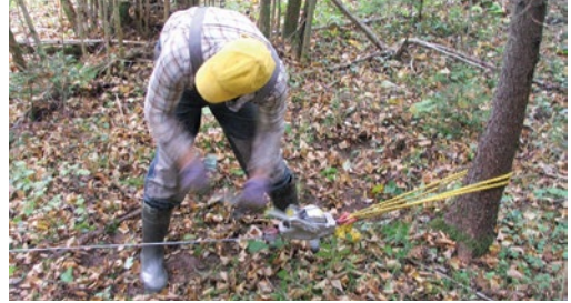
A hand pulley is used for the removal of large dimension wood from rivers with steep banks inaccessible for machinery. Photo: A. V. Urtāns.
