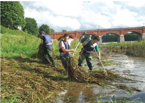
Manual withdrawal of macrophytes. Before pulling them ashore, macrophytes are left to drain of water for several seconds for easier transfer. R. Venta. Photo: A. V. Urtāns.
