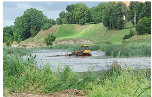
Use of caterpillar tractor on shallow dolomite ground for creation of a riffle. R. Mūsa. Photo: A. V. Urtāns.
