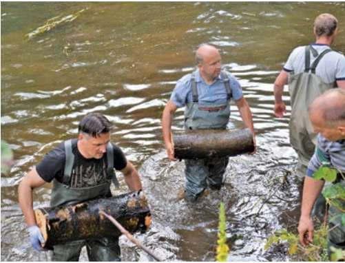
Timber logs are sawn in dimensions that can be lifted manually. R. Svētupe. Photo: Ē. Kļaviņa.
