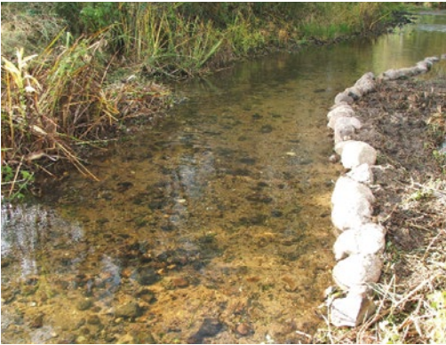
Rows of stone promote narrowing of the stream, and sediment scouring. Photo: L. Urtāne.
