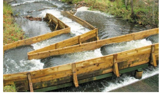
Fig. 17.36. Cascade-type fishway in the River Līgatne. Photo: A. V. Urtāns.
