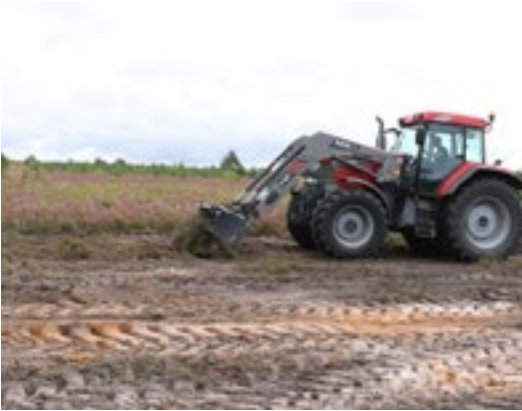
Fig. 18.16. Topsoil removal with front loader and bucket. Ādaži military training area. Photo: I. Mārdega.
