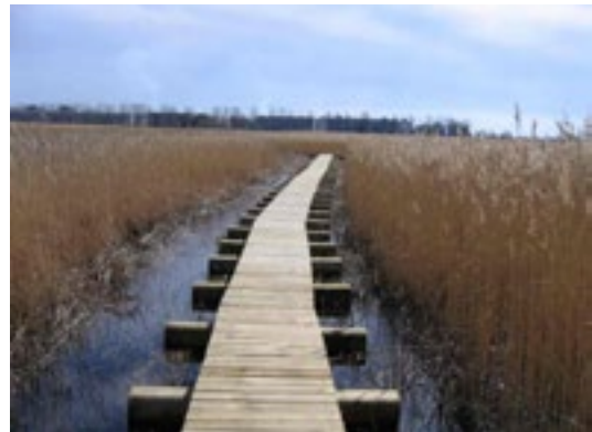
Fig. 10.19. Boardwalks raised above the water level save habitats and help to organise recreation and the education of people. Daugavgrīva, "Piejūra" Nature Park, 2006. Photo: B. Laime.
