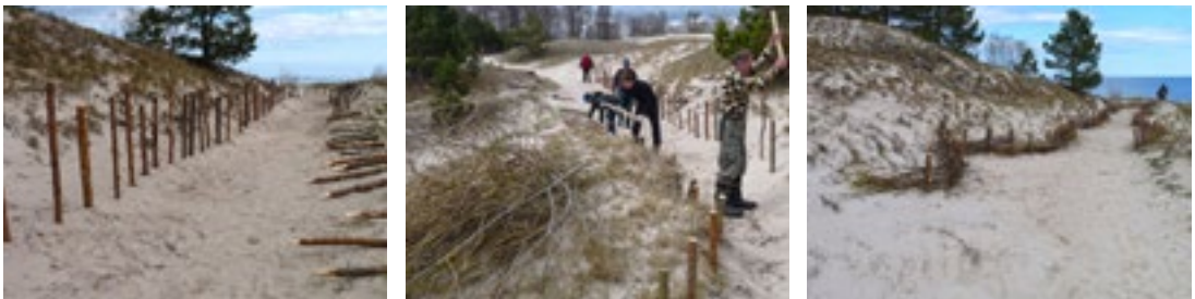
Fig. 14.49. Fence construction of twig wickerwork, Nature Reserve “Pliņciema kāpa”. Grey dune and foredunes are protected from intense trampling. Year 2011. Photo: K. Lapiņš.
