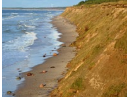
Fig. 12.6. Relatively slow formation of vegetation on a sea cliff slope of fine-grained sediments; north of Jūrkalne (six years since the erosion episode). Photo: J. Lapinskis.
