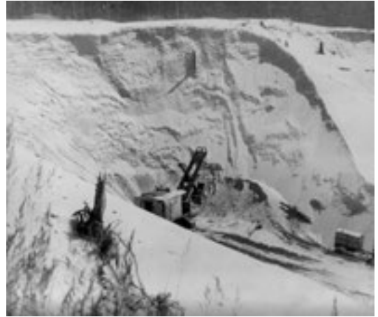
Fig. 2.9. The excavation of White dune in Bernāti in the 1960s. Photo from the archives of Gita Vanaga.
