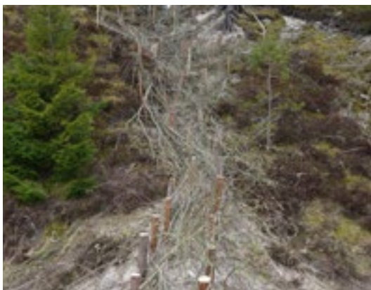
Fig. 13.15. Use of dune covering with branches is one of the most cost-efficient methods for dune restoration and coastal sand habitat strengthening. Ķemeri National Park, years 2011 and 2005. Photo K. Lapiņš, B. Laime.
