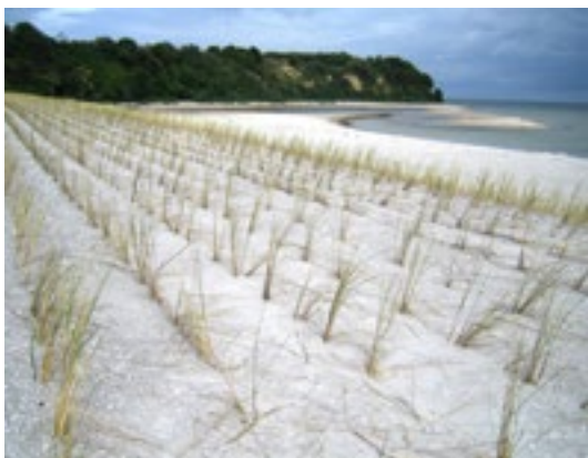
Fig. 13.20. Dune sand strengthening with grass planting. Germany, 2010. Photo: K. Vilciņa.
