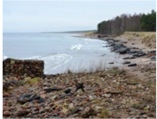
Fig. 12.13. Coastal erosion intensification nearby the coastal section protected by an anti-erosion structure, at Liepāja wastewater treatment plant. Photo: J. Lapinskis.
