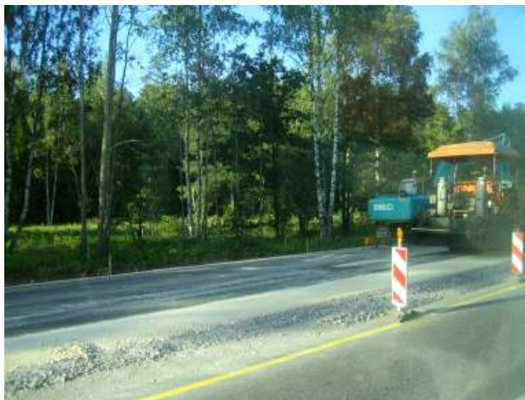
Enlargement works on A-2 by the NP.
