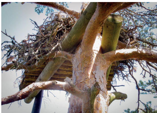
Klinšu ērgļa aizņemta mākslīgā ligzda. Platformas balstiem izmantoti virpoti, impregnēti mieti. Foto: J. Ķuze. Artificial nest, occupied by Golden eagle. Nest supports are built from turned and impregnated sticks. Photo: J. Ķuze.
